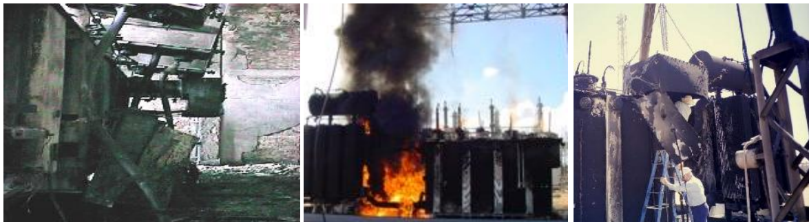
a) Burnt out transformer after a 132kV cable termination failure. b) Transformer fire caused by 11kV cable termination failure c) Cable box after fire. Cables & gland plate blasted off by arcing fault
