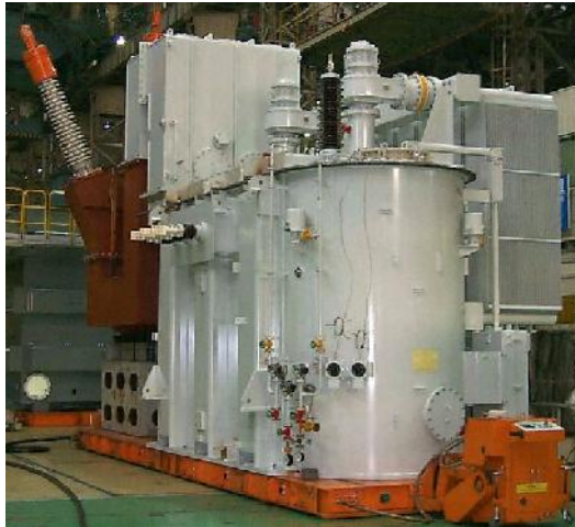
a) Low Pressure GIT 110kV-50MVA
