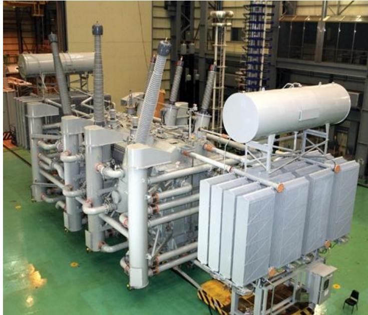
Figure 18: Transformer equipped with a 40 rupture discs depressurization system
