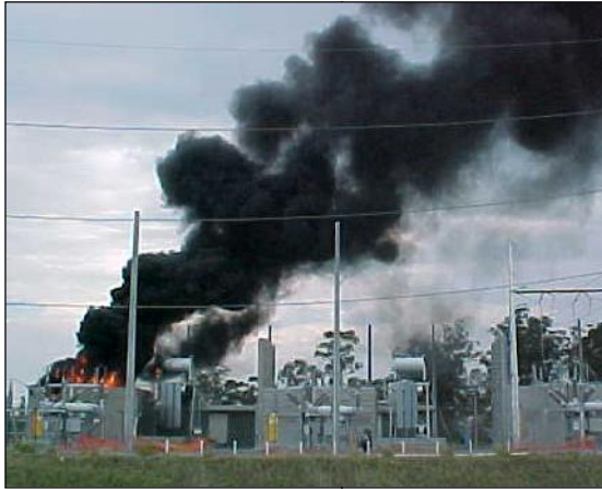
Fire contained to 1 of 3 transformers
