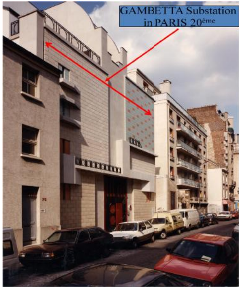
Exterior View. As can be seen from the picture the substation blends in well with the street-scene, with the only noticeable difference being the fairly wide access door
