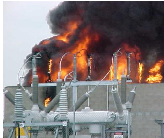
Fire contained to within sound enclosure. Polymer SA insulators on top of enclosure wall only melted on side towards fire only. HV Switchgear remained intact.
