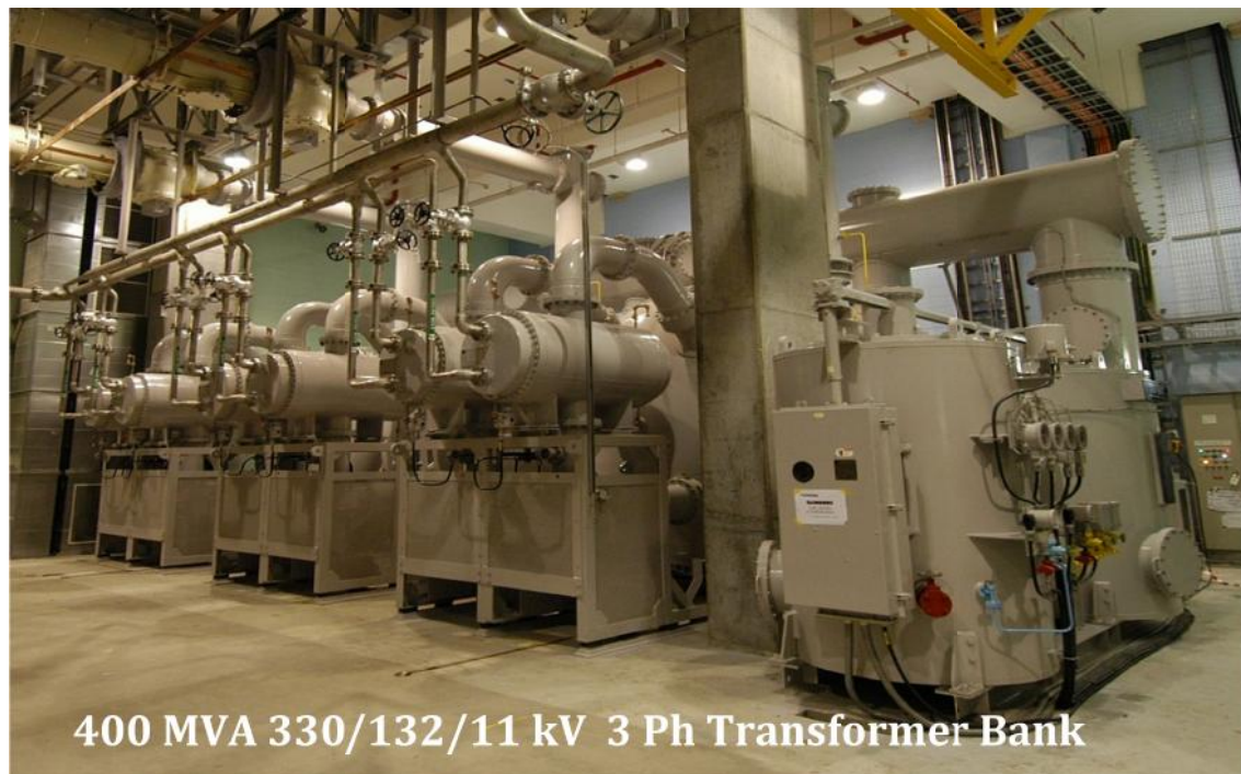
Figure 60: SF6 underground substation in Sydney [63]
