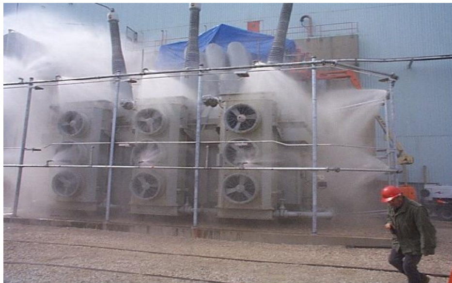
Figure 54: Water spray system with rock filled pit
