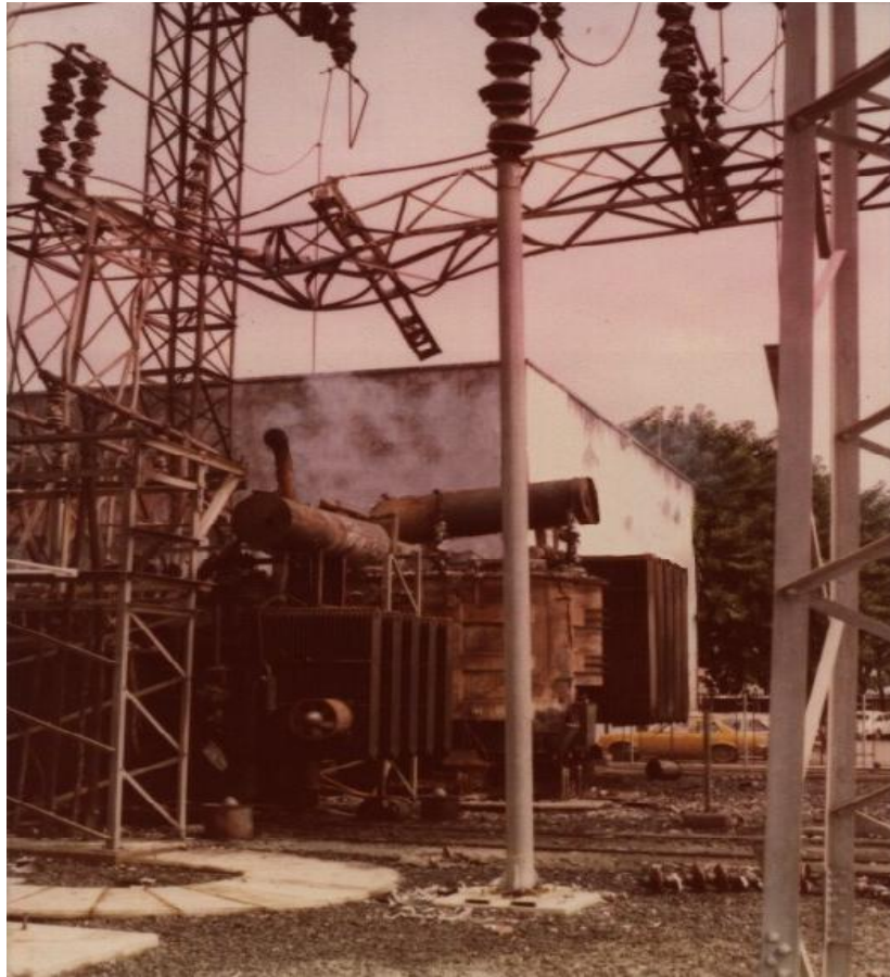
Figure 28: Deformation of the High Voltage Landing Span Structure after a Transformer Fire
