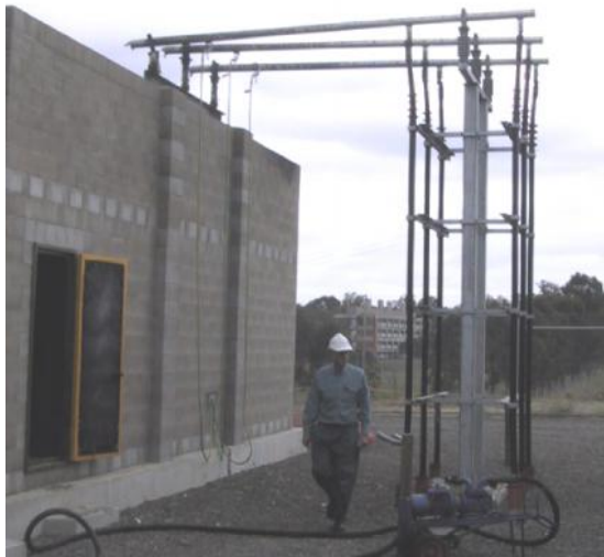
Aluminium busbar partly melted, but secondary cables and cable terminations intact.
