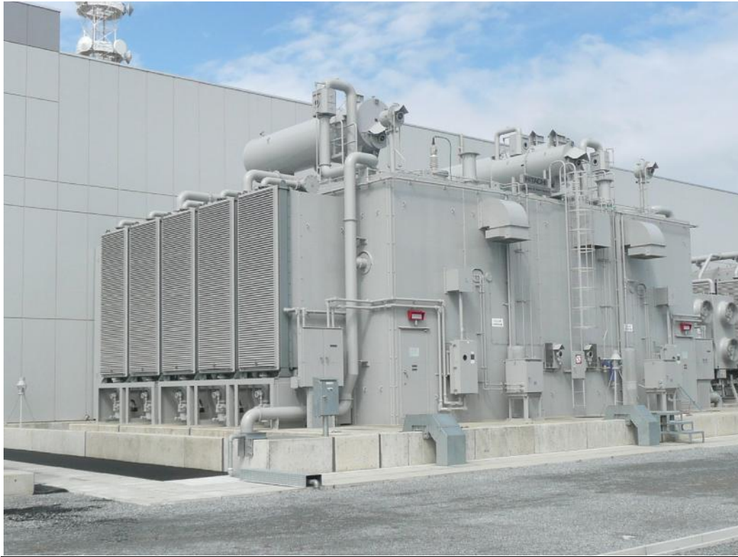
Figure 58: Fire Suppression system using inert gas on transformers installed within sound enclosure panels
