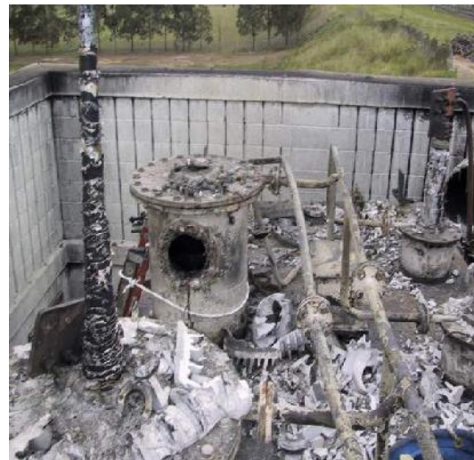
Top of transformer the day after
