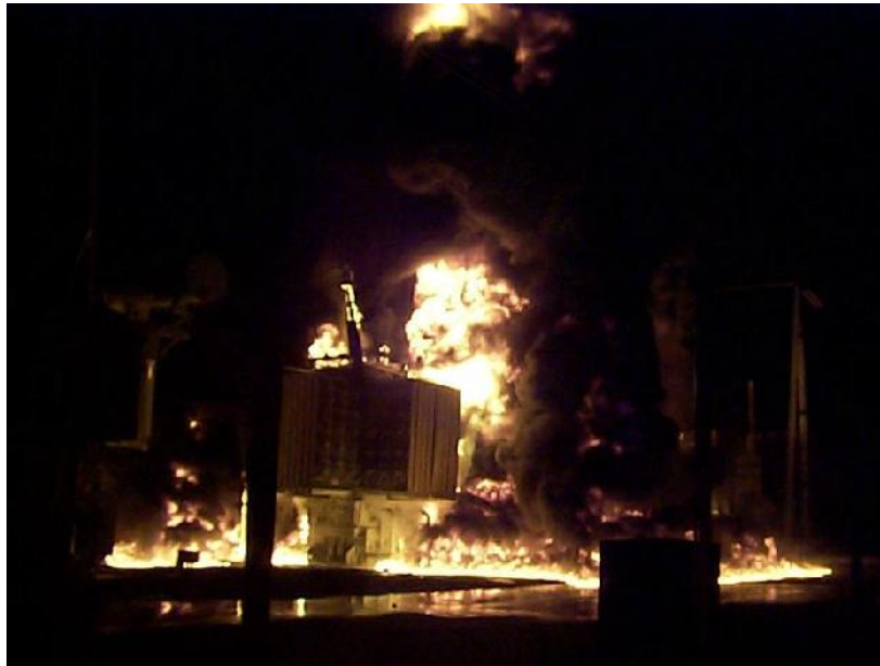
Figure 25: A transformer involved in a pool fire
