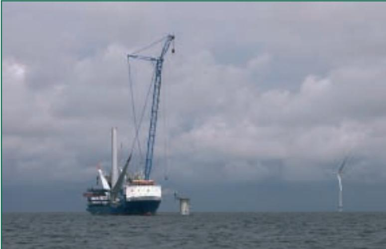
Figure 2. Offshore assembly of wind generators with a crane mounted on a special ship (Courtesy Vestas Central Europe)
